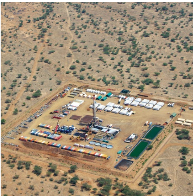
Drilling at Amosing discovery, Kenya
