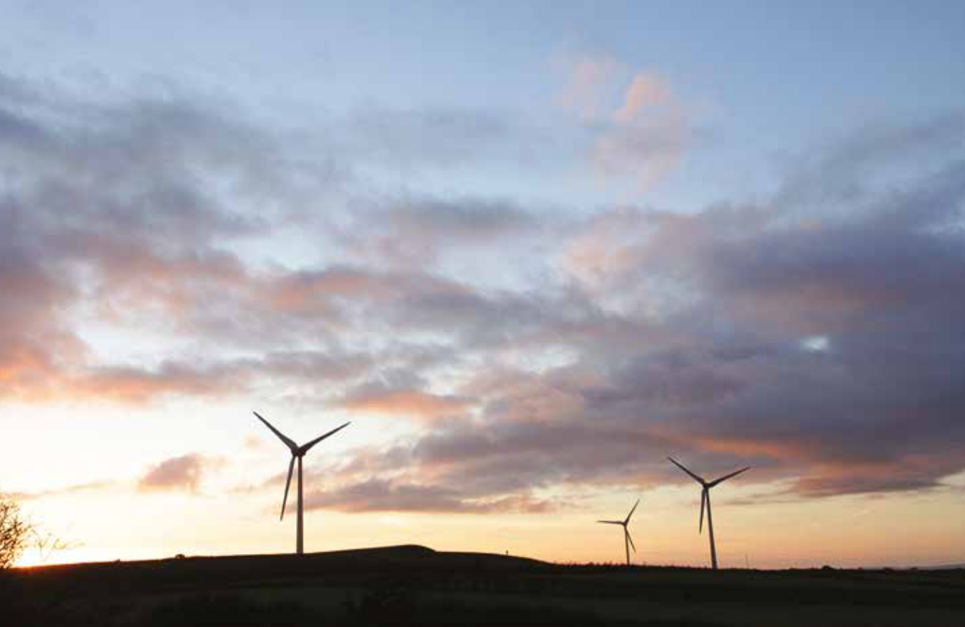
Dusk falls at Delabole wind farm, Cornwall.
