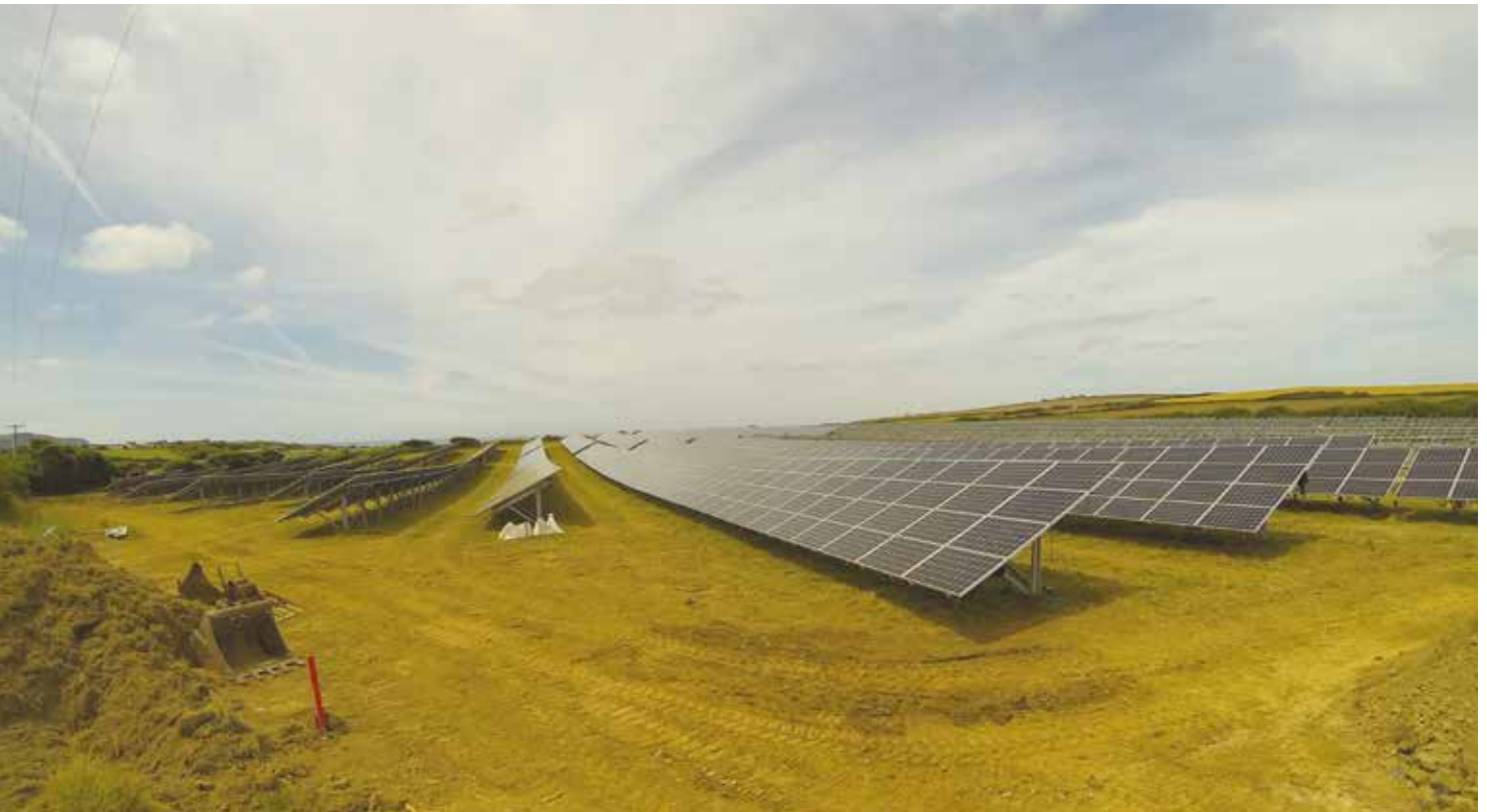
Good Energy's solar site at Creathorne Farm, north Cornwall, was commissioned in the summer of 2014.
