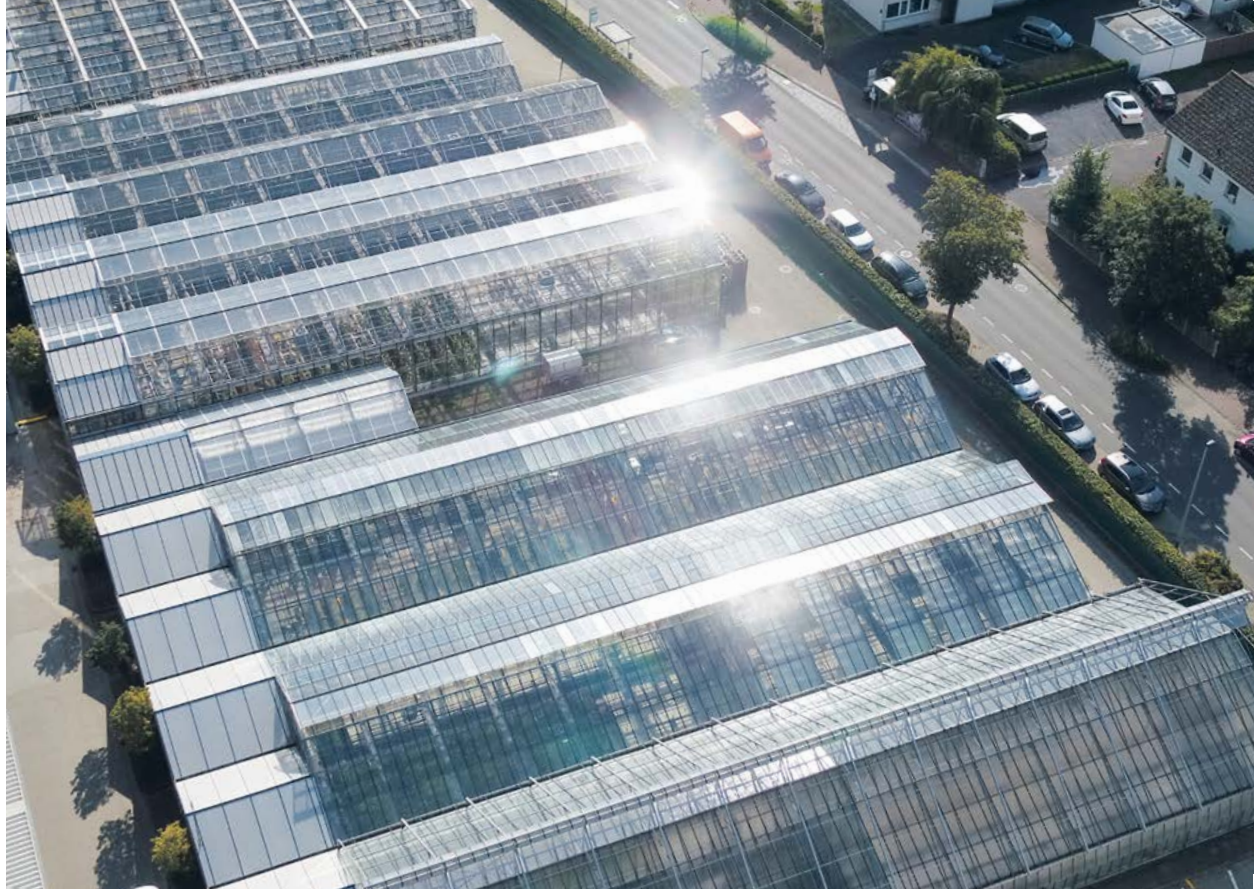
Greenhouses and climatic chambers not only need heat, but cold too. The recently completed new central cooling plant in Einbeck ensures that energy is produced more efficiently and distributed better across the campus.
