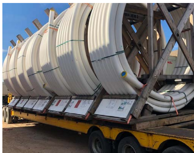
Rolls of composite pipe used to repair flowline connecting MB-2 well to the Mnazi Bay gathering system
