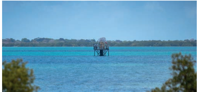
Refurbishment of MB-1 Well Platform
