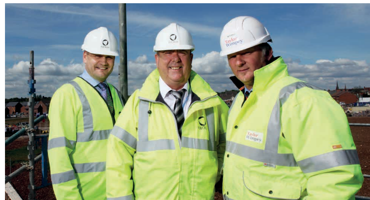
Regional Operations Manager, Martin Peters and Field Officer, Mick Hill on site with Taylor Wimpey Site Manager Mick Wale
