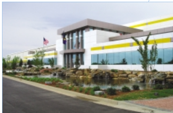
Fred's new distribution center in Dublin, Georgia. Opened April 2003.
