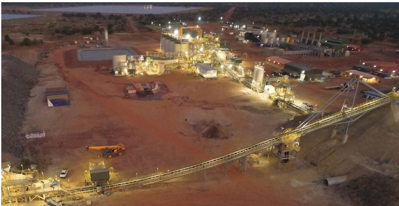
figure 4 – Sanbrado process plant
