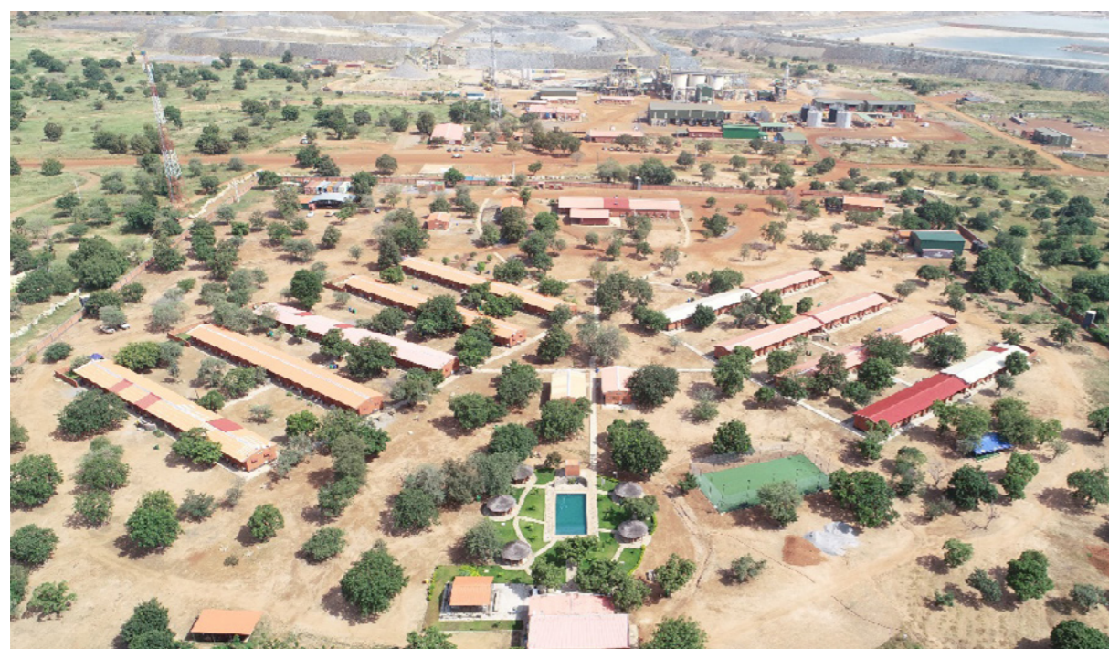
FIGURE 5 – SANBRADO ACCOMMODATION CAMP WITH PROCESS PLANT IN BACKGROUND
