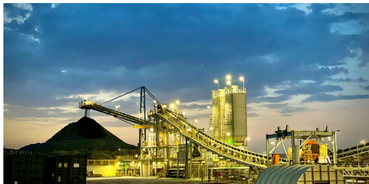
FIGURE 4 – SANBRADO PROCESS PLANT
