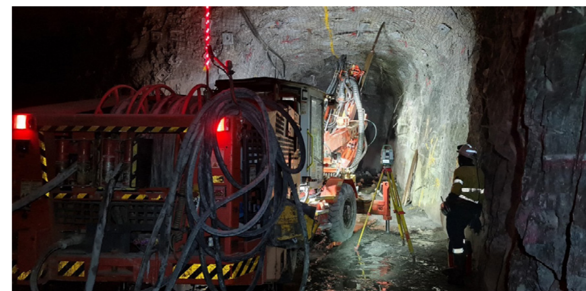
FIGURE 3 – INSTALLING MESH AT M1 SOUTH
