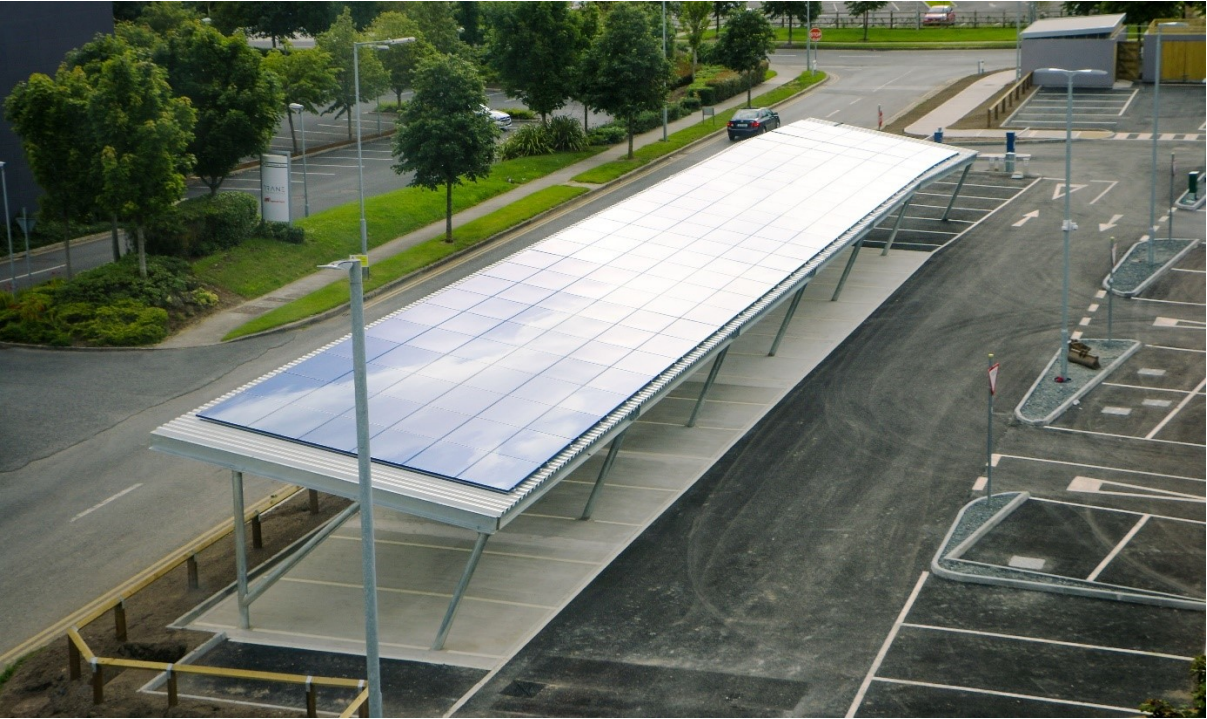
Solar panels at Ryanair's Dublin Campus
