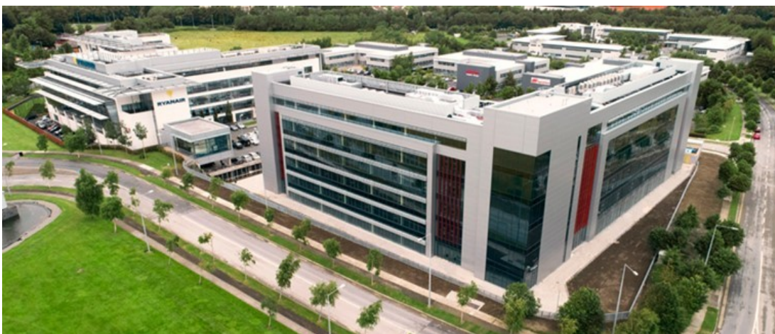
Ryanair's Dublin Campus at Airside Business Park, Dublin, Ireland
