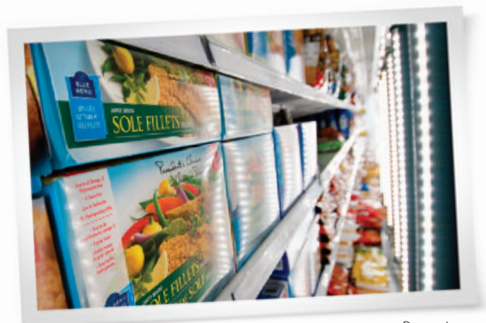
Motion-activated LED lights at Scarborough Loblaw Superstore.
