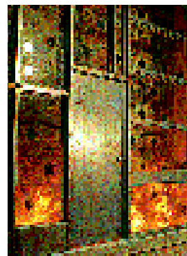
Fire-resistant steel doors made by Curries and fire doors with wood paneling produced by Graham prevent the spread of fire while allowing time for safe evacuation.
