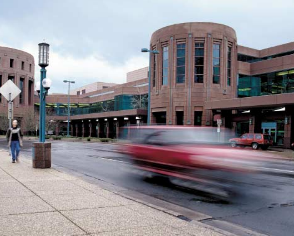
The new addition to the Minneapolis Convention Center combines the solid traditional security of a SARGENT mechanical key system with a SECURITRON digital entry system and exit delay system. Exit delay systems secure exterior doors electronically while permitting authorized entry, but delay unauthorized egress from within, so reducing loss from theft.
