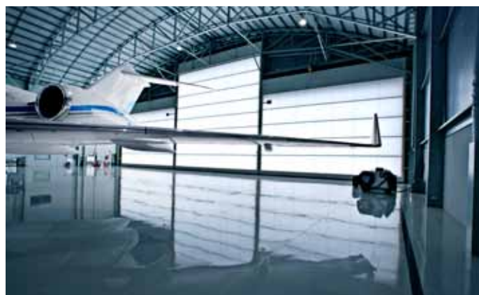
Megadoor hangar door.
