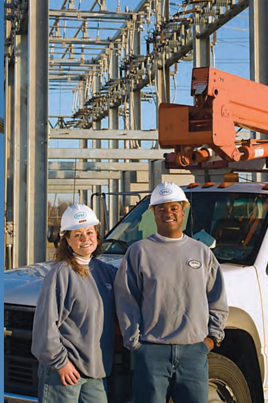
Allison Coate (left) and Quintin Gaddis play a valuable role in substation construction. DP&L built three new substations during 2006 to strengthen reliability and supply power to the region's growing areas.
