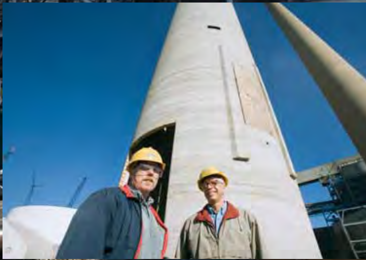
Wendell Adkins (left) and Earl Bush are part of the DPL team managing the $500 million scrubber installation project. The new 800-foot stack at Stuart Station will contain four flues, one for each of the four generating units at the plant.
