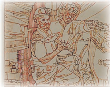
A Tait Station turbine being repaired by Ted Wilks (left) and Willie Davis.
