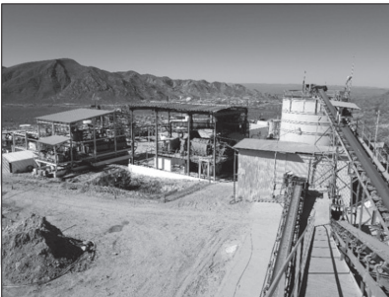
VELARDEÑA PROPERTIES - OXIDE PLANT
