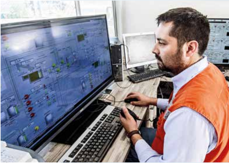
Fibre optic cable technology is already being used at our operations in Chile to enable near-real-time measurement and monitoring of tailings dam conditions, including structural movements, seepage levels and the degree of settlement taking place. Featured in the control room at Los Bronces' Las Tórtolas operation is tailings dam operator Carlos Onetto.
