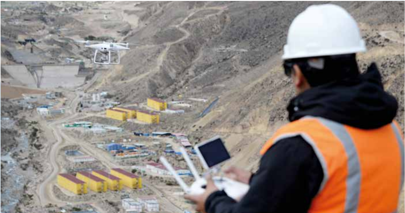
The use of drone or Unmanned Aerial Vehicle (UAV) technology, across a number of our mining activities, is helping to contribute to the successful delivery of our FutureSmart Mining™ programme. Drones, or UAVs, can be used for a number of activities, such as supporting safety and hazard management, generating images, measuring production performance and to evaluate mining conditions.
