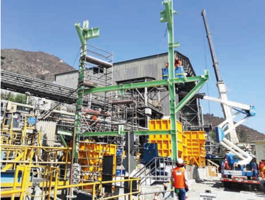
Construction of the Hydrofloat™ pilot-scale plant at El Soldado in Chile.
