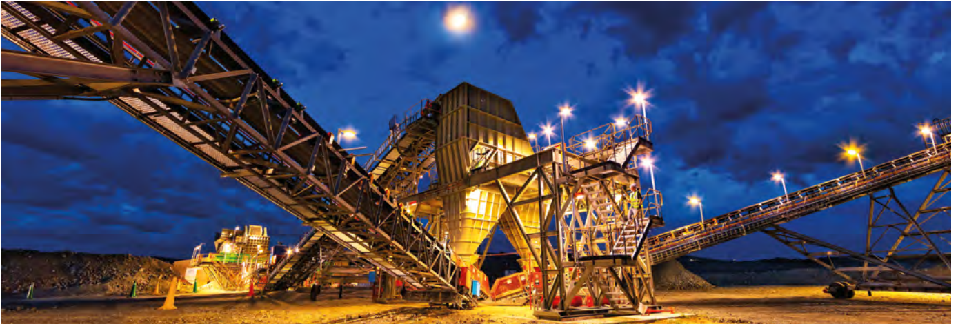
⤴ Bulk ore sorting (BOS) plant at PGMs' Mogalakwena mine. The BOS system unlocks production capacity through early rejection of waste, reducing the volume of material sent to the processing plant.
