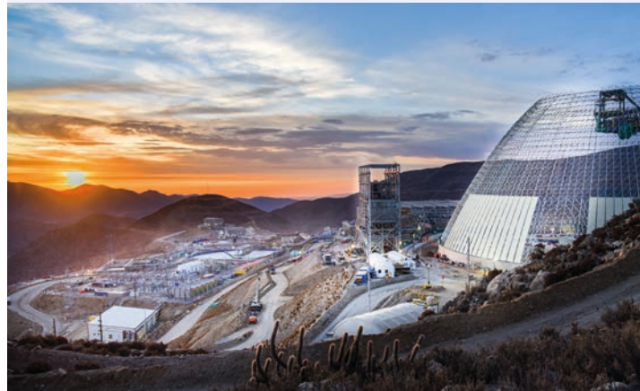
▲ Construction work in progress at Quellaveco's futuristic-looking Papujune processing plant.
