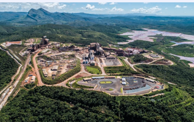
▲ The Minas-Rio mine site in Minas Gerais, Brazil.
