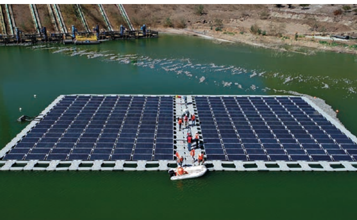
▲ This photovoltaic (PV) facility, built over a tailings pond, supplies solar energy to power the new hydrogen plant at Las Tórtolas, part of the Los Bronces mine complex in Chile.
