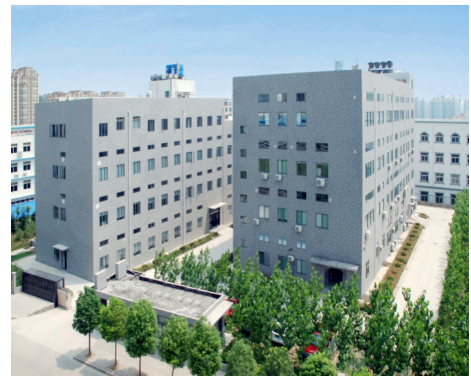
Hefei Co-source Bio-medical Co. Ltd building Shushan District, Hefei, Anhui, P.R China.
