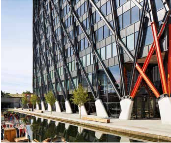
Brunel Building W2 – completed in May 2019
