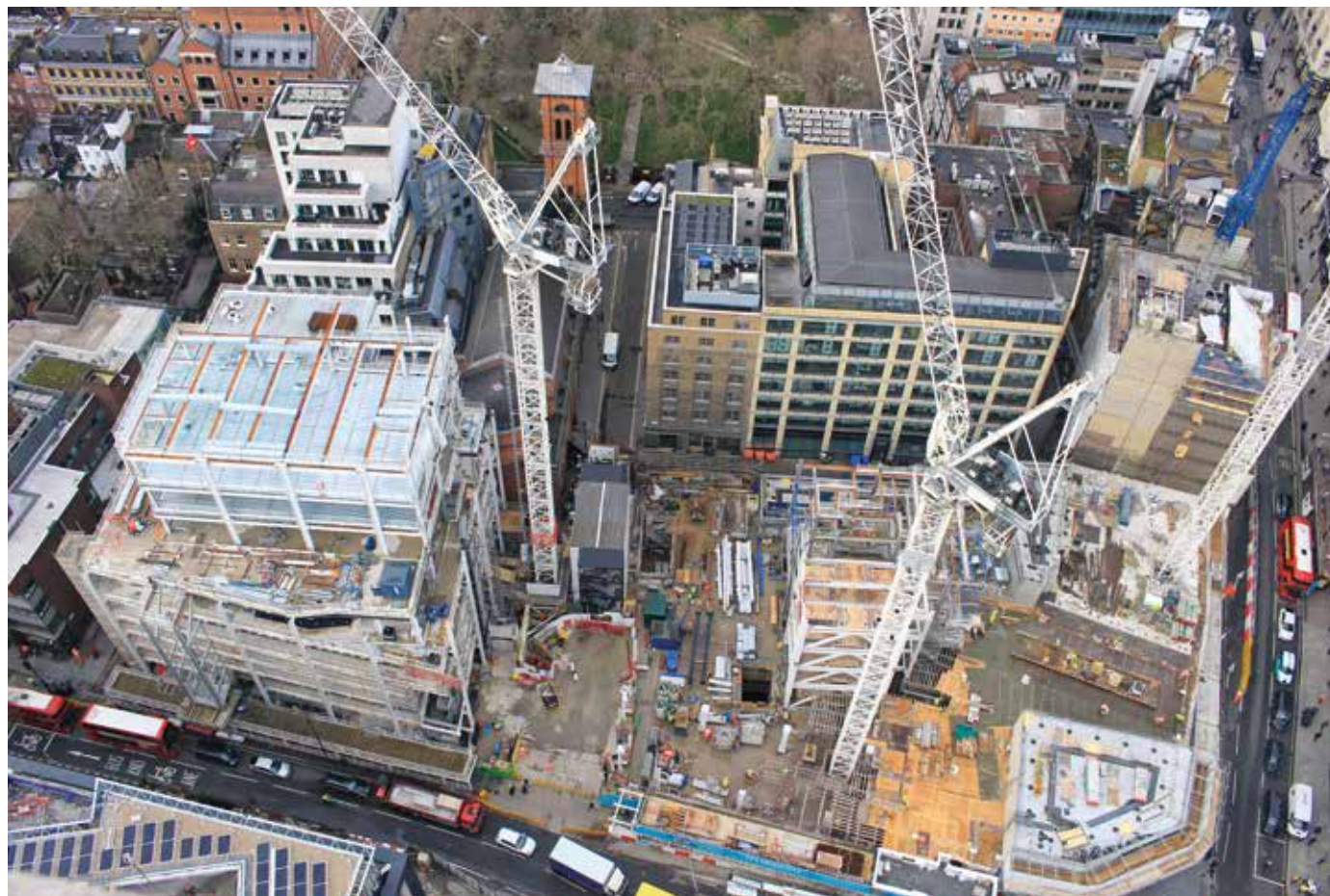
Soho Place site
