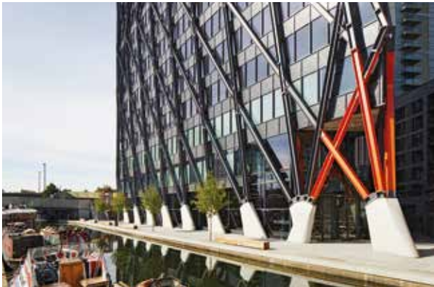
Brunel Building W2
