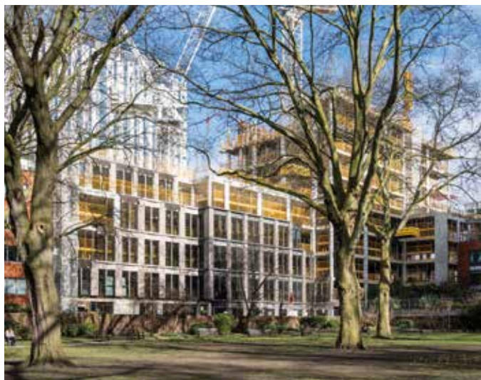
The Featherstone Building EC1 – Early payment to our subcontractor Skonto Plan (based in Latvia) for the façade cladding enabled our main contractor Skanska to store the majority of the façade elements before 31 December 2020. This meant site operations were able to continue unaffected by tariffs and the movement of goods arising from Brexit.
