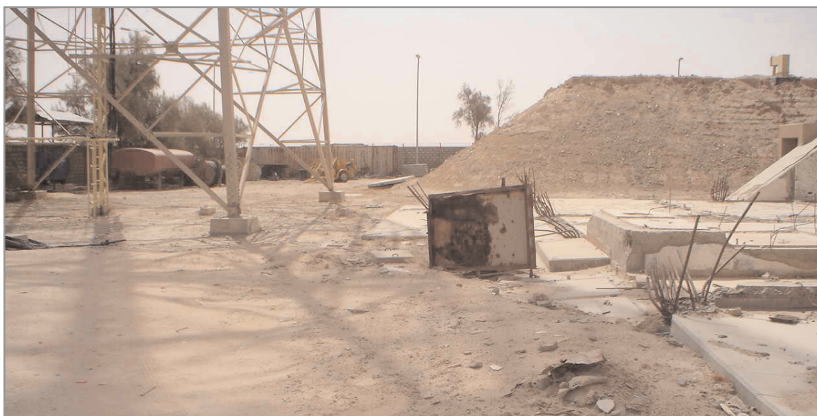
Figure 8: PS1 Oil Receiving Station Q4 2008 (Subba and Luhais)
