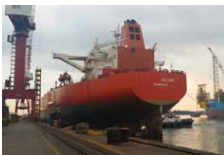
Kraken FPSO under construction.
