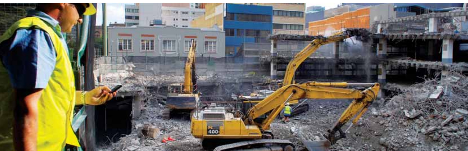
Development underway at 123 Albert Street, Brisbane
