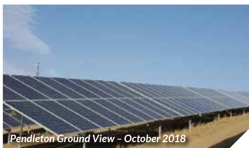
Pendleton Ground View - October 2018
