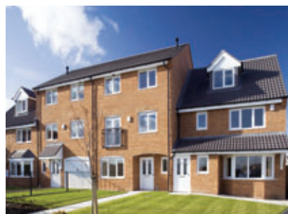
▲ Herons Reach, Barnsley, South Yorkshire.
