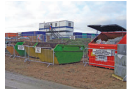
▲ Bellway compound showing recycling and waste segregation.
