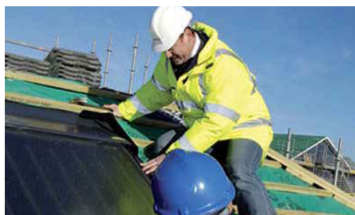
Solar panel installation, Cleadon Vale, Tyne and Wear.
