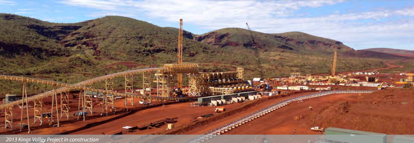
2013 Kings Valley Project in construction
