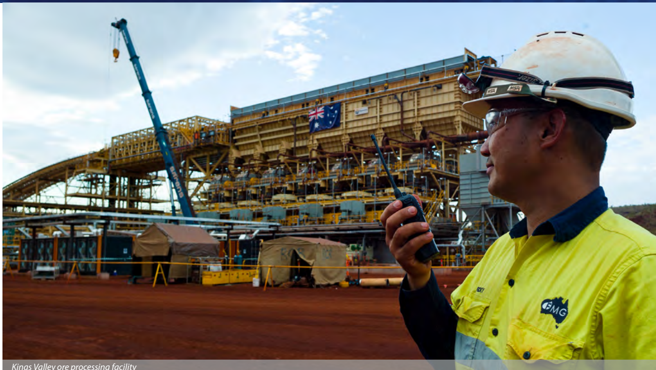
Kings Valley ore processing facility
