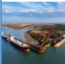
Anderson Point Berth 5 completion Fortescue River Gas Pipeline completion
