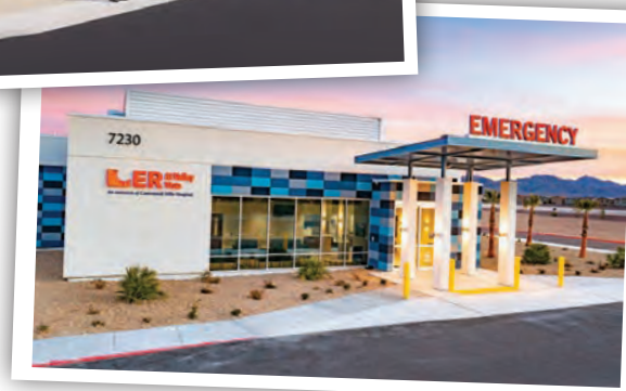
ER at Valley Vista, an extension of Centennial Hills Hospital Medical Center
