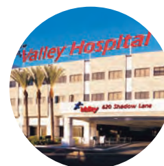
Valley Hospital Medical Center
