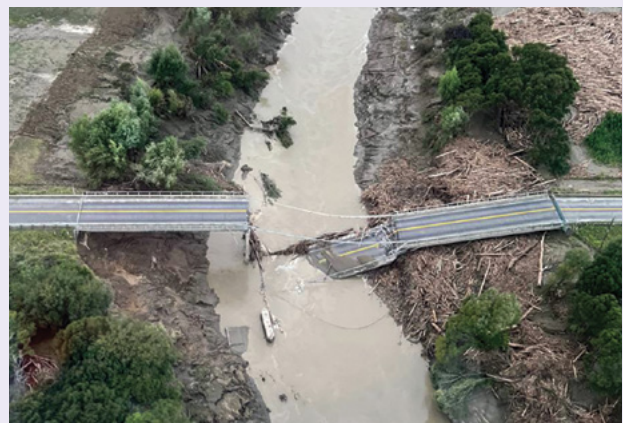
Damage to the regional fibre route on the bridge crossing the Hikuwai River, north of Gisborne, required 800 metres of fibre to be overlaid.
