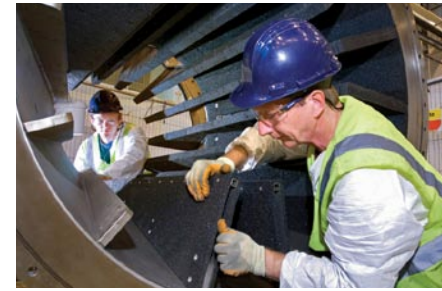
Above, through a U.K. subsidiary, our Electronic Technologies Group supplies the Rutherford Appleton laboratories with resin-bonded boron carbide neutron shielding panels at the ISIS accelerator in Oxford, England. The Electronic Technologies Group has deep experience in such niche products.
