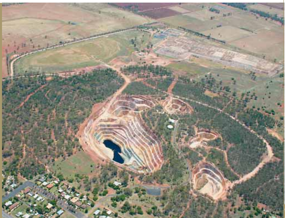
Peak Hill Gold Mine – pit and heap leach pads
