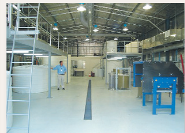
DPP main shed
