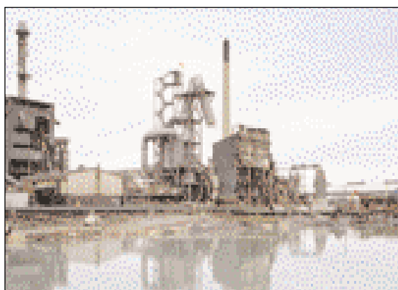
Demolition in progress at Britannia Zinc, Avonmouth.
