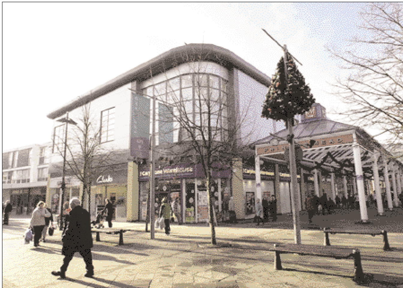
The Mead — an initial phase of redevelopment, completed and let during the year at Farnborough, Hampshire.
