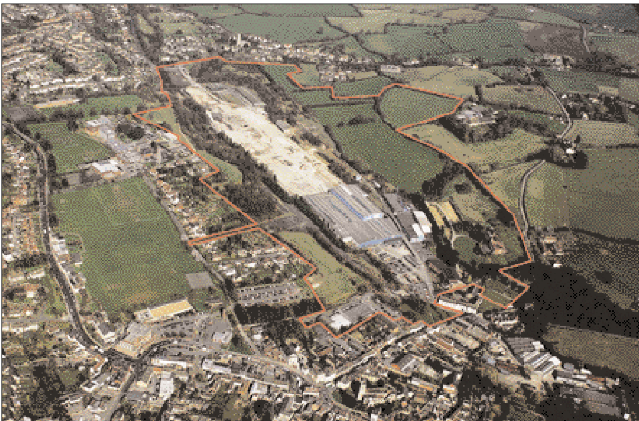
A 92-acre former manufacturing site being redeveloped as an urban village at Dursley, Gloucestershire, in joint venture with SWRDA.
