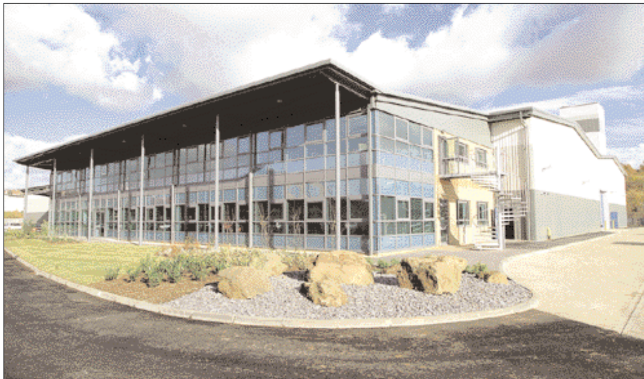
A 70,000 sq. ft. industrial building constructed for Mapei at Coombs Wood, Halesowen on a 43-acre former steelworks site developed through a joint venture with Corus plc.
