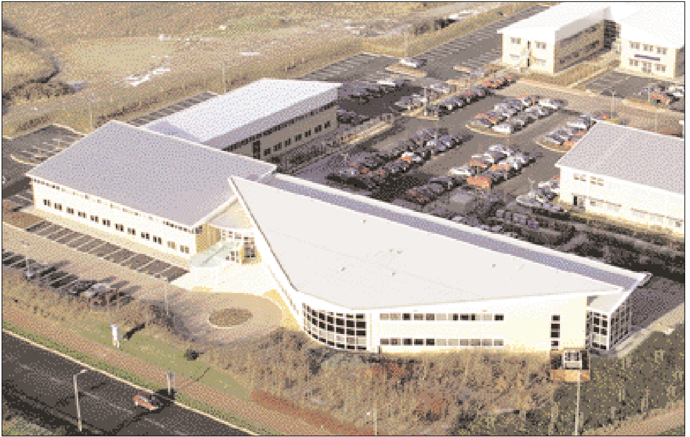
Cranfield Technology Park, a joint venture with Cranfield University, where we manage 77,000 sq. ft. of high tech/office space on flexible leases.
