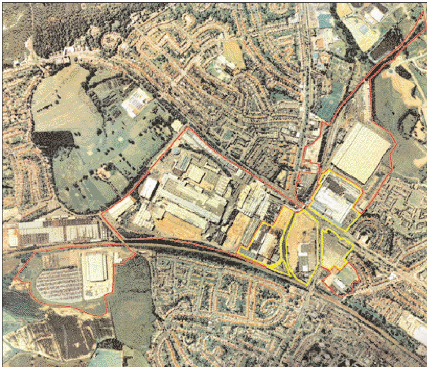
Longbridge, Birmingham: 228 acres (edged red) — acquired and leased back to MG Rover in December 2003. 40 acres (edged yellow) — appointed as developer by Advantage West Midlands.
