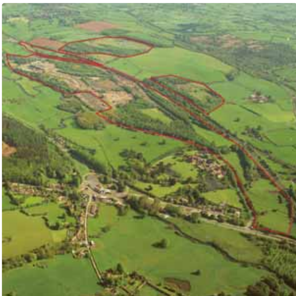
Meaford Power Station: 100 acre site acquired in the year.
