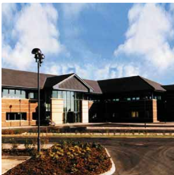
Quinton Business Park: 25,000 sq.ft. building let to the Highways Agency and sold during the year.
