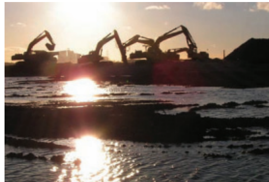
◀ LLANWERN EARLY REMEDIATION WORKS TAKING PLACE ON THE SITE
