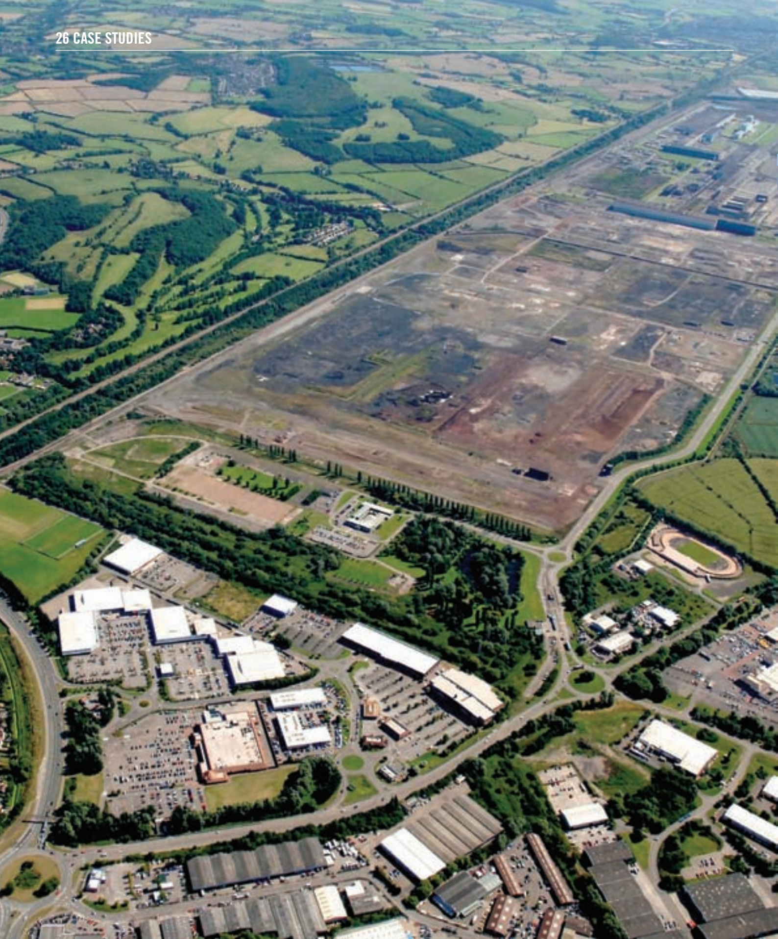
▲ LLANWERN A 600 ACRE MIXED USE DEVELOPMENT, FOR WHICH PLANNING PERMISSION HAS BEEN OBTAINED. INFRASTRUCTURE WORK TOGETHER WITH THE FIRST RESIDENTIAL PHASES WILL COMMENCE IN 2008
