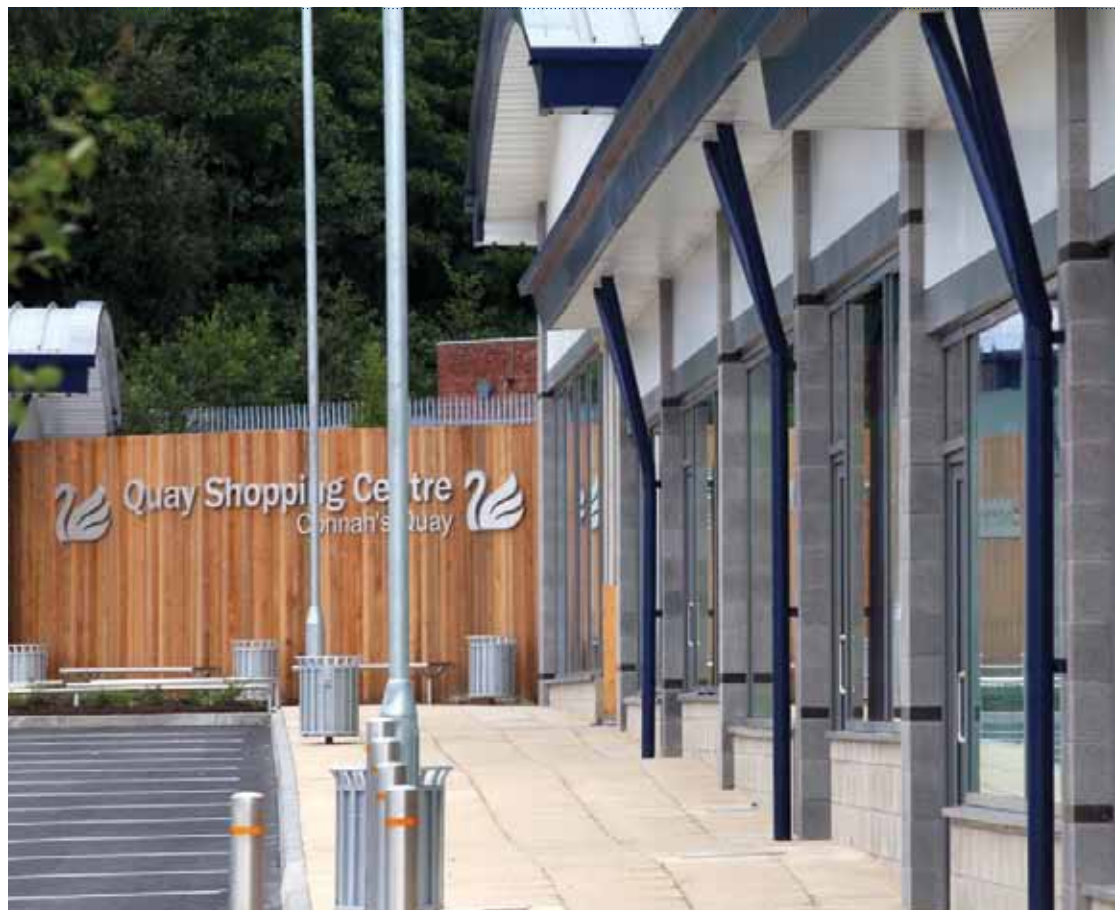
← The completed 52,000 sq. ft. Morrison's foodstore at Connah's Quay, Flintshire. This is part of our Quay Shopping Centre development.
