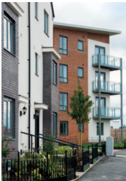
Above: Akron Gate, Goodyear, Wolverhampton, a scheme of 453 units and built by Persimmon as part of our joint venture.
