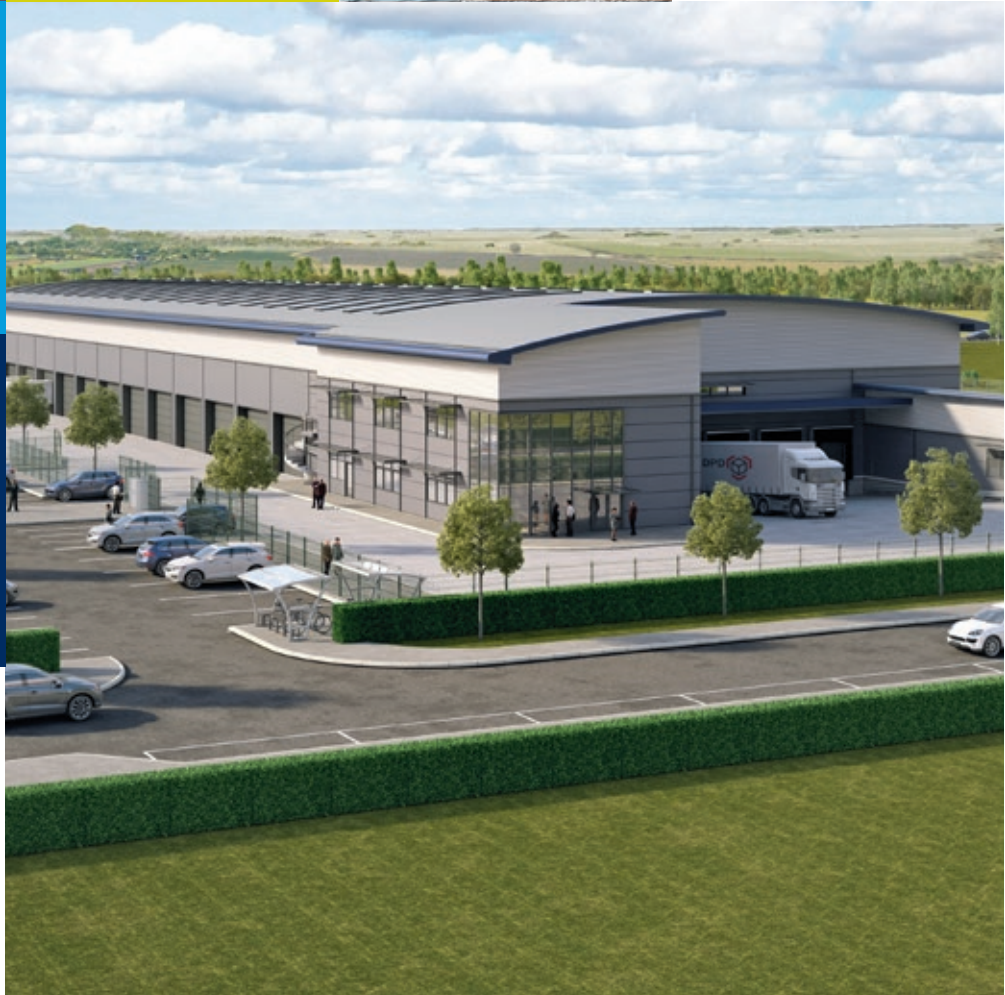
PICTURED RIGHT: Our Skypark project in Exeter will deliver 1.4m sq ft of office and industrial manufacturing space, including a 60,000 sq ft distribution centre for DPD (UK).
