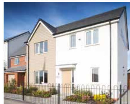
Above St. Modwen Homes is progressing well with the first phase at Meon Vale.
