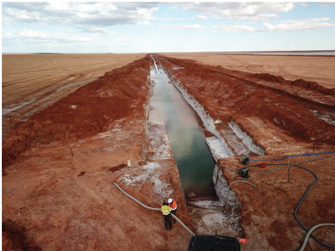
Figure 6: 3.4km Trench providing additional brine to Lake Way Evaporation Ponds
