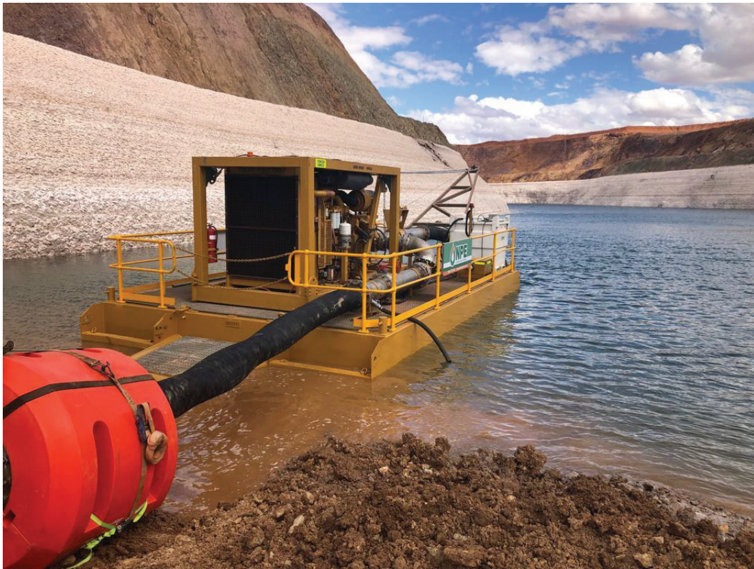
Figure 5: Dewatering of Williamson Pit
