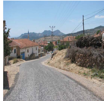
Paved village roads near Kışladağ
