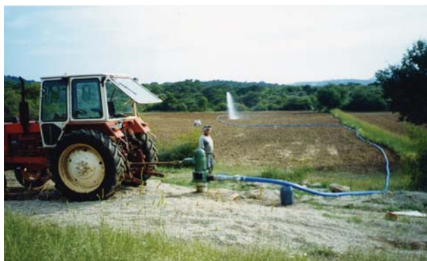
We constructed new agriculture water wells to provide water for crops in the area surrounding Perama
