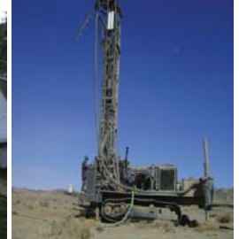
Rotary Air Blast Drilling
