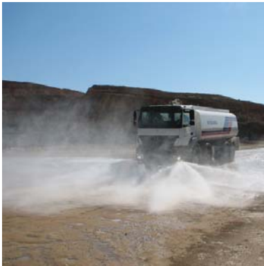
Dust control on mine roads at Kışladağ
