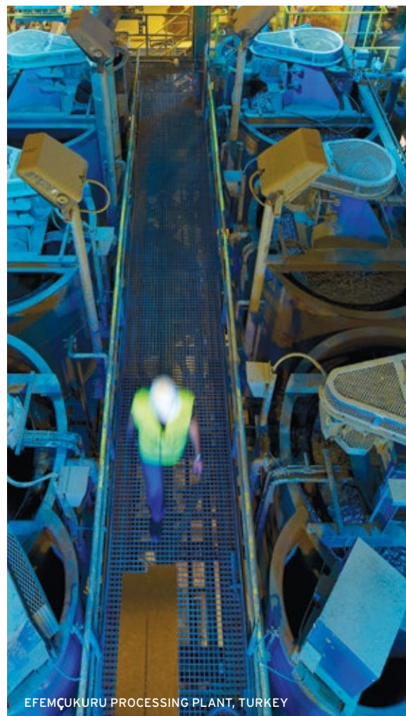
EFEMÇUKURU PROCESSING PLANT, TURKEY
