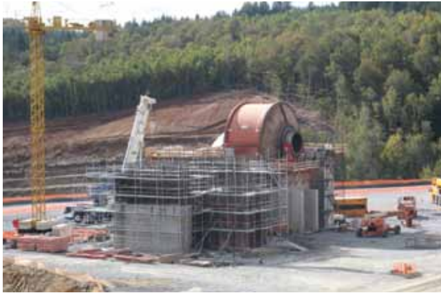
Installation of the SAG mill at Skouries, Greece
