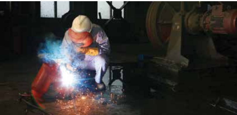
Welding at Tanjianshan, China
