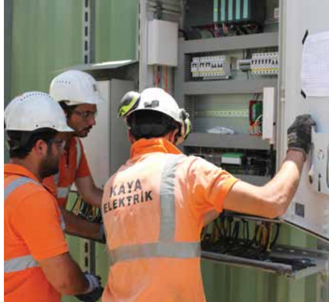
Local electricians work at Efemçukuru, Turkey
